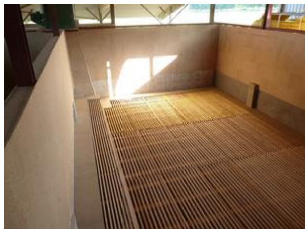
Figure 7 : Séchoir couloirs (MOPINET, 2020)
